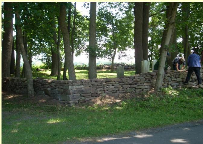
The photo shows the reconstruction of a portion the northwest corner of the wall surrounding the Reading Burying Ground in Rosemont. Additionally, the south west corner has since been repaired. The cost was well under the estimate of \$4000. Look for a full photo report on the MTAP web site in the future.
