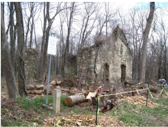
Early work in progress
